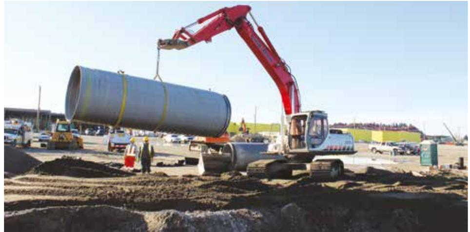
**A 6-metre-long section of large diameter SaniTite HP pipe is moved into place. The polypropylene pipe provides the additional stiffness plus the long bell and dual gaskets needed to compensate for the area's soft soils.**
