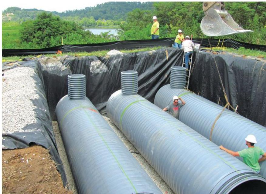
A Worthington, Ky., project sought to minimize sanitary sewer overflows into the Ohio River with 860 ft of 60-in.-diameter pipe installed in a three-row configuration.
